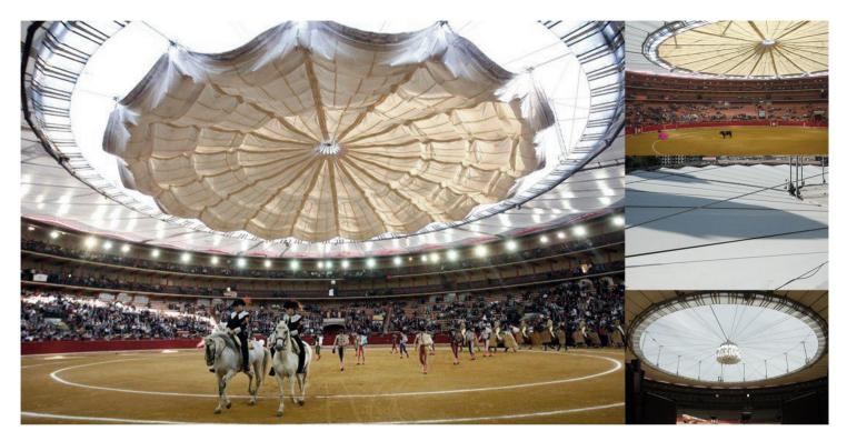
The structure of the existing roof consists of a fixed part and a mobile section in which the structural resistance is conferred to a system of cables which is anchored in a perimeter beam which acts as a compression ring that rests upon a system of column supports.
